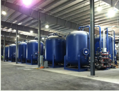
WATER TREATED Completed
